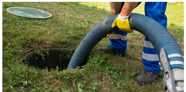
Pumping out a septic tank
