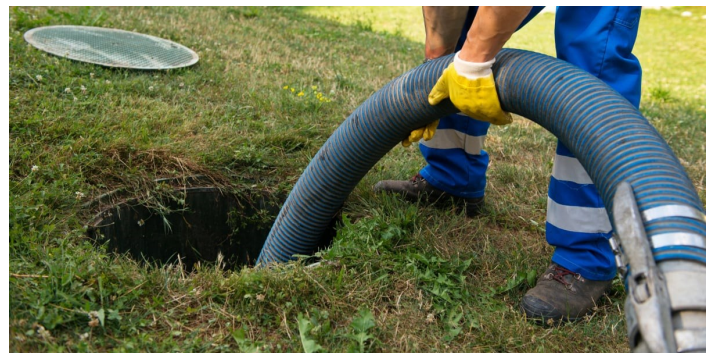
Pumping out a septic tank
