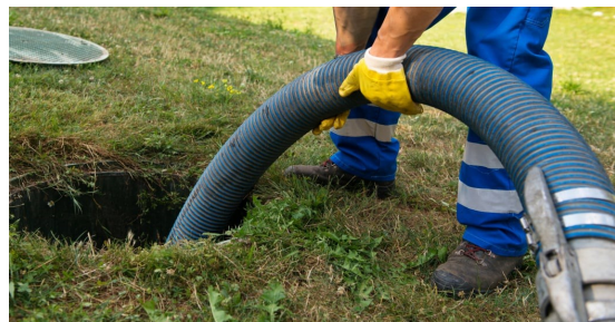
Pumping out a septic tank
